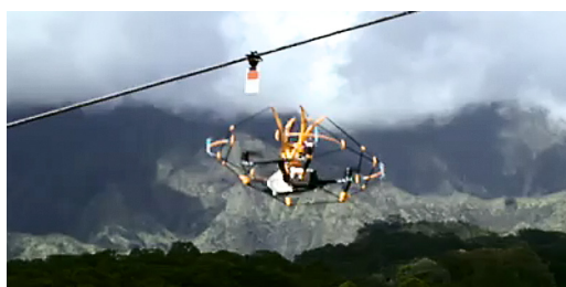
FireFly diverters can be installed by drone
