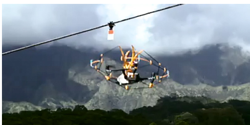
FireFly diverters can be installed by drone
