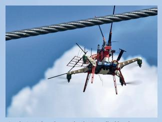
FireFly & BirdMark can also be installed by drone.
